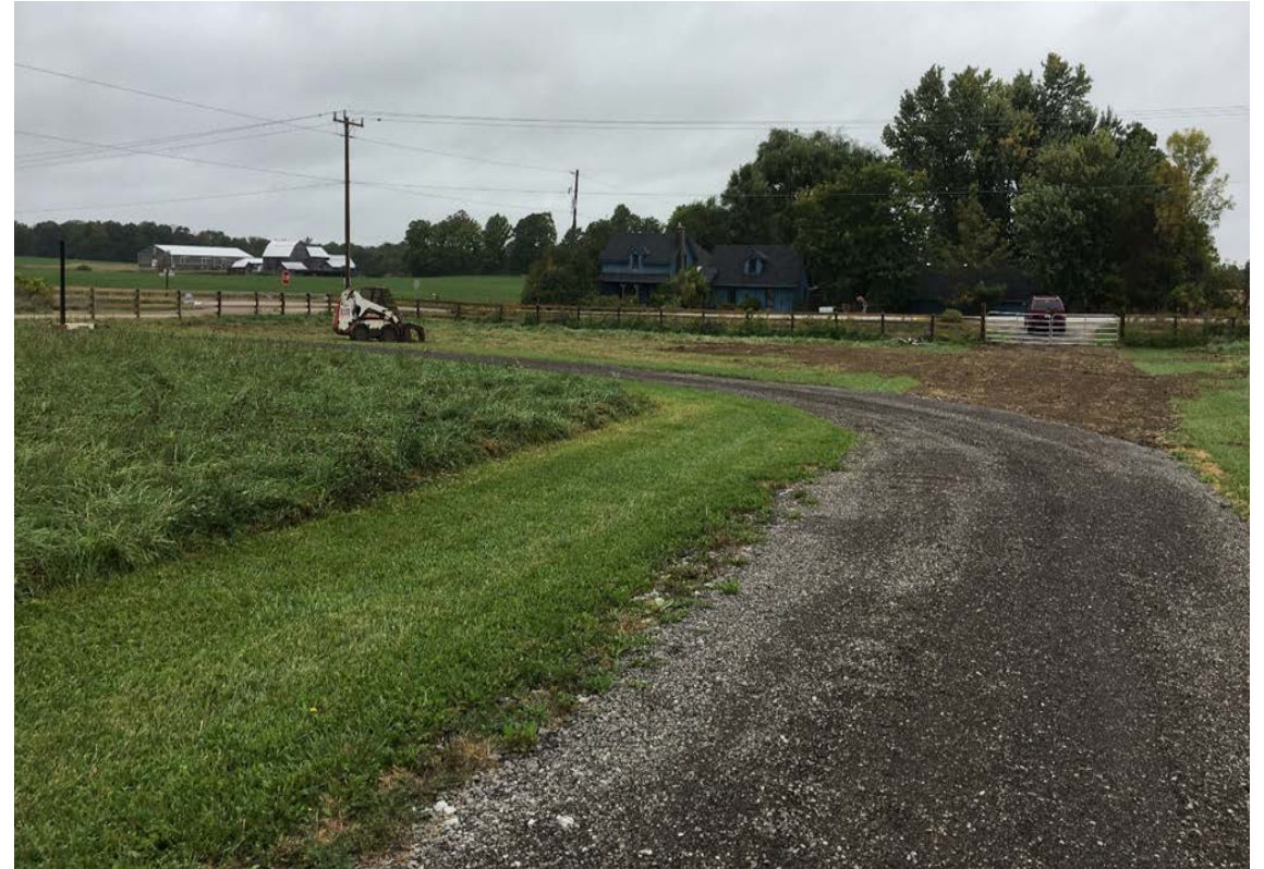
ORMLT/OFT CEA Little Rock II with the rerouted driveway; restoration plan with additional vegetation planned for spring 2019
