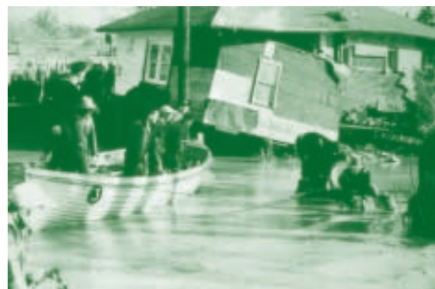
Hurricane Hazel – flood damage and rescue
